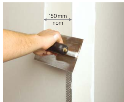
2. Apply first coat to both corner faces
