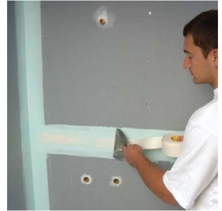
3. Bed in paper jointing tape at sheet joints.
