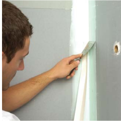
2. Bed in paper jointing tape in the corners.
