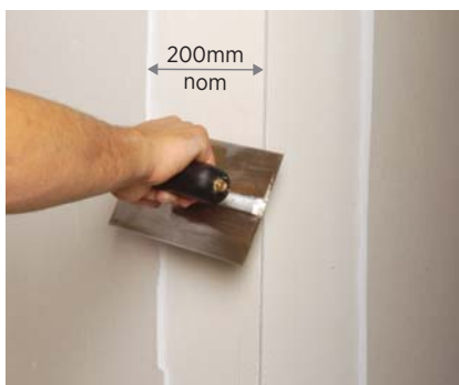
3. Apply second coat to corner faces
