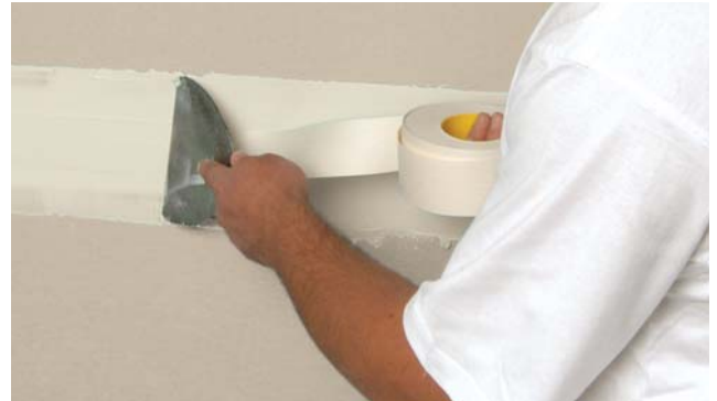
2. First coat - Bed tape
