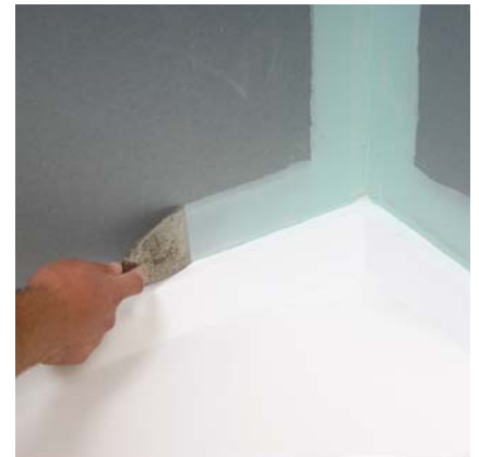
6. Apply skim coat of Wet Area Taping Cement at sheet base.
