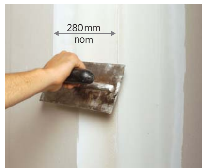
4. Apply third coat to corner faces
