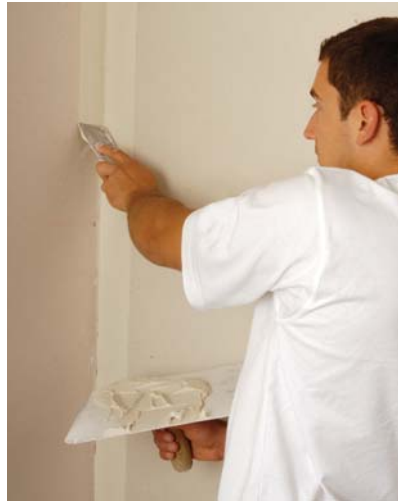
1. Apply base compound
