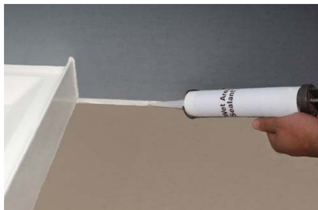
Figure 61: Seal Floor and Wall Junctions
